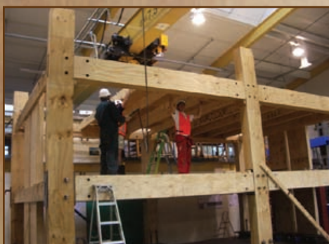
Pre-fabricated post and beam construction for buildings up to five storeys tall.
