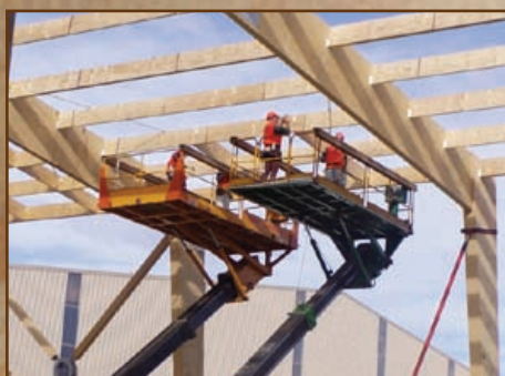
Single storey warehouse type buildings, incorporating large open spans.
