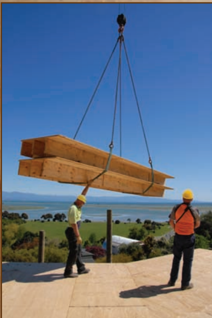
Potius Floor Panels span up to 11m and boast rapid installation and light weight.
